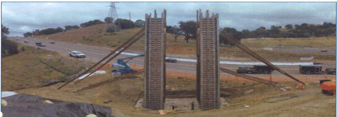
45' single-lift concrete formwork and bracing
