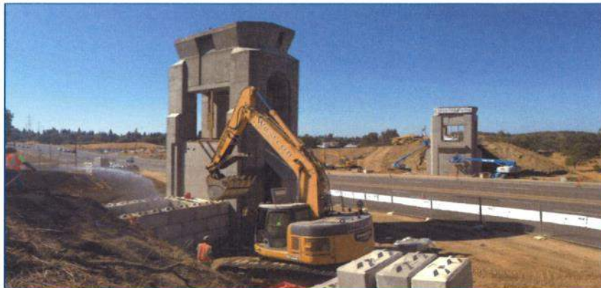
UltraBlock abutment and approach walls under construction
